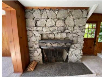
Interior - First floor fireplace
