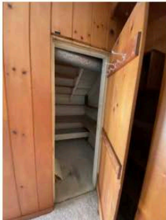
Interior - under stair storage closet
