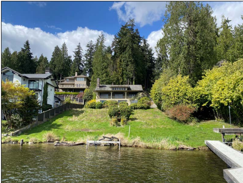
Figure 17. Overview of the eastern half of the project in the vicinity of probe #2, 3, and 4. View to the west.
