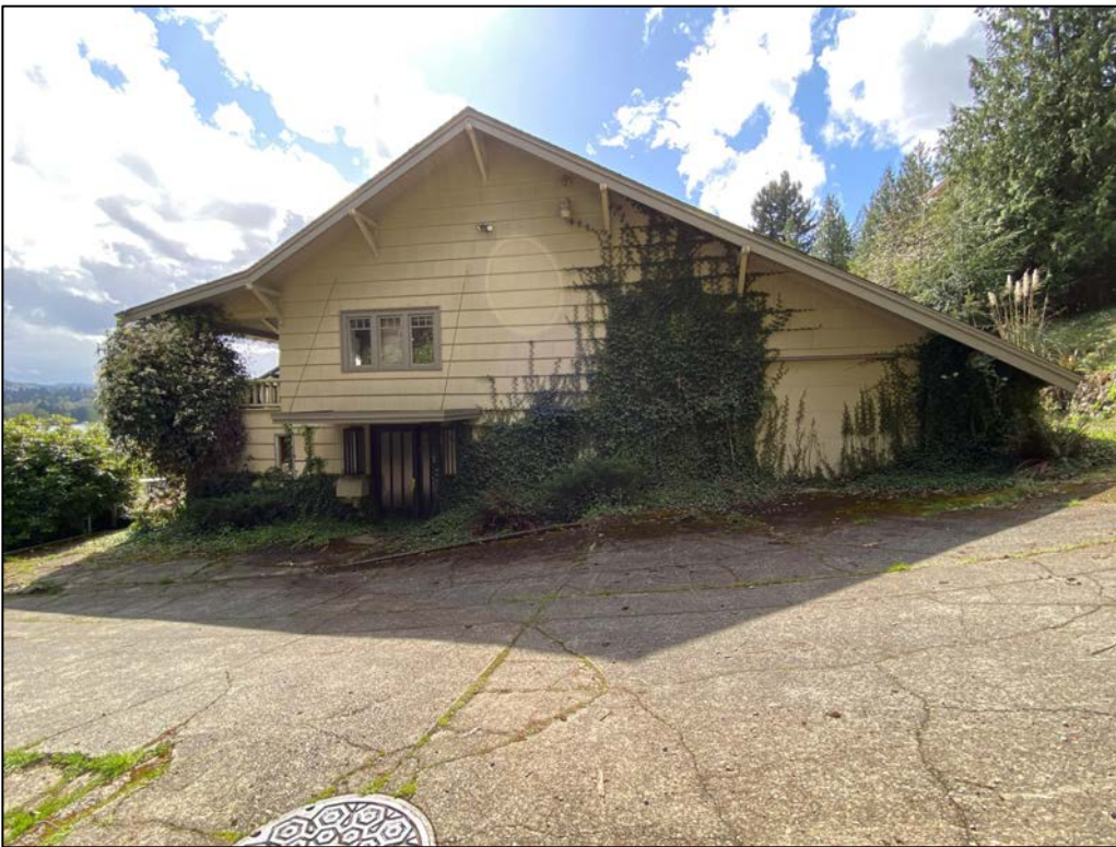
Figure 19. Overview of the northern half of the project in the vicinity. View to the south.
