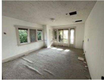
Interior - Northeast secondary bedroom
