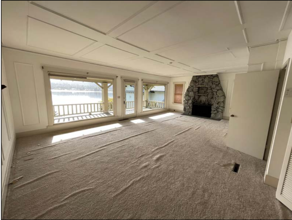
Figure 28. Image of the main bedroom, showing the rough-cut stone-clad fireplace, molded picture frame paneling, full-light single-entry door, picture windows, and forced air registers at the entrances. Image taken from the closet, view to the southeast.
