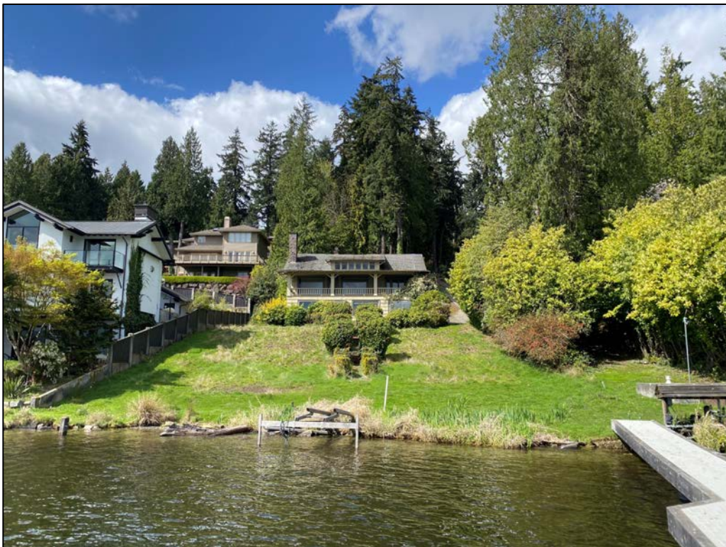
Figure 25. Overview of the ca. 1908 single-family residence and associated secondary structures at 4006 E Mercer Way (DAHP Property # 283025). Image taken from the boat slip on the dock, view to the east.
