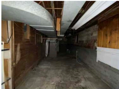
Interior - Unfinished first floor/basement
