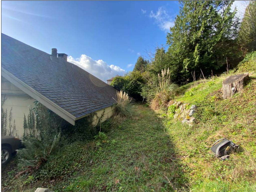
Figure 21. Overview of the western half of the project and in the vicinity of probe #1, View to the south.
